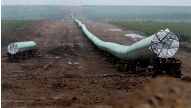
*This is a portion of the new 42-inch natural gas pipeline being installed near Alpine, Texas. This portion of the pipeline is just north of Alpine. The pipeline starts at the town of Coyanosa and will extend 148 miles just 12 miles upriver from Presideo, Texas.*
